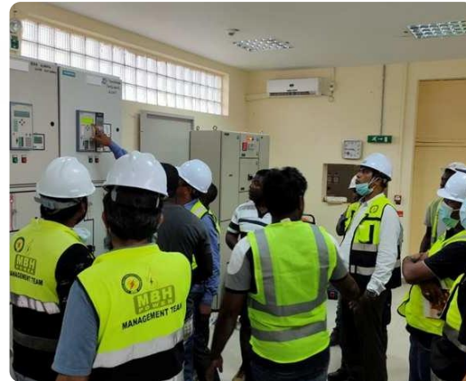
● Charging the Lines
